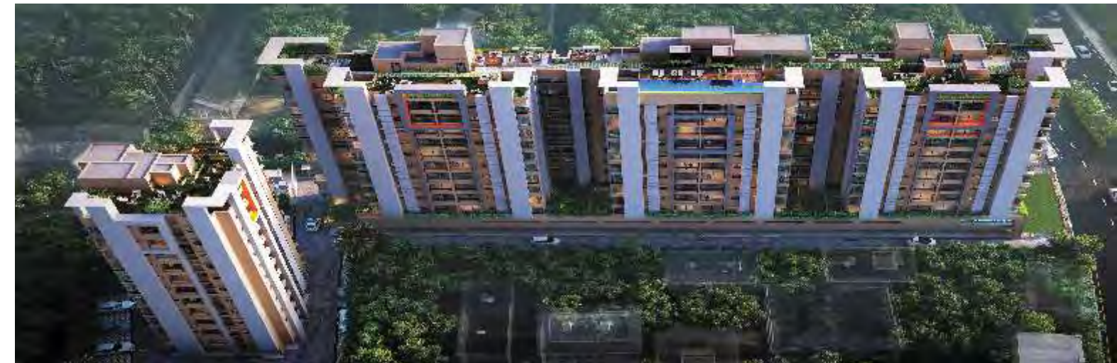
RISHI VENTOSO, Madhyamgram, Kolkata (Under Construction)
