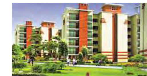
RISHI APARTMENTS*, Baddi, Himachal Pradesh
