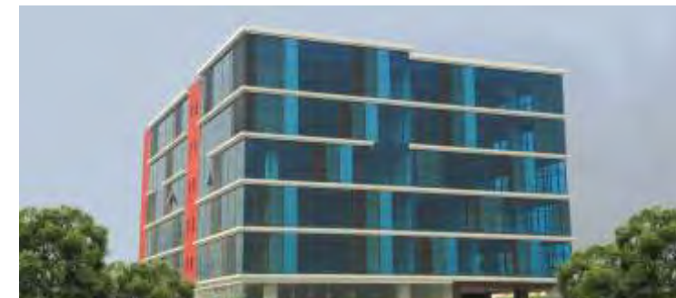
RISHI TECH PARK, New Town, Kolkata (Delivered)
